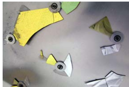
Fig. 5. Collector fragments still attached to array frame. Compare fasteners to Fig. 1 pre-flight.
